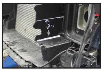
21. Using the utility knife, cut a piece 3" wide from the middle of the corrugated plastic. This will allow the baseplate to slide on.
